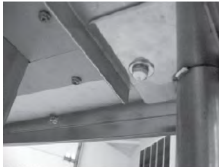
Figure 2-6 HHS Bolts Secured
